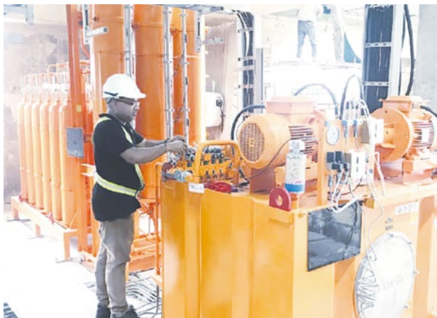
Commissioning Engineer working on Governing System Oil Sump tank at Da Nhim Hydro Project site in Vietnam
